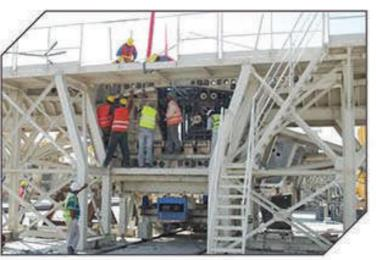
Finalizing position of ducts inside segmented section of bridge prior to pouring concrete.
