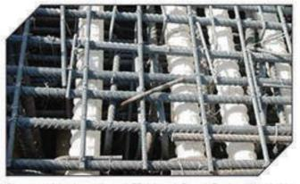
Close-up of body section of PP Internal Round Ducts resting inside segmented section of bridge - BEFORE pouring of concrete.
