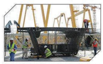
Early stage of placing ducts in appropriate positions inside segmented section of bridge.
