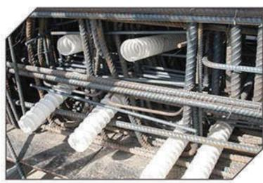
Close-up of end section of PP Internal Round Ducts resting inside segmented section of bridge - BEFORE pouring of concrista.
